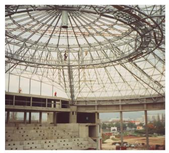
Figure 21. Partial view of the roof from the assembly period
